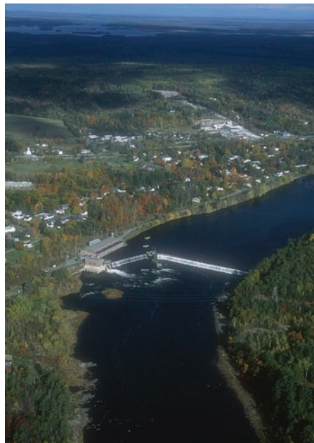
The Veazie Dam would be removed as part of the Penobscot project. (Photo: Heather Perry)
