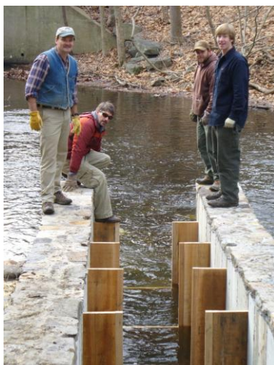
SG, Tim Wildman, Dave Ellis and seasonal Gabe Luongo pose for photo after inserting the last weir into the fishway last fall. (photo by Sally Harold, TNC)
