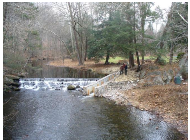
The Low Dam (named for the owner not the height) and the pool-and-weir fishway to the right, as observed from the downstream bridge. (photo by SG, CTDEP)
