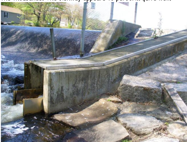
A side view of the Gorton Pond Fishway, showing the entrance.
