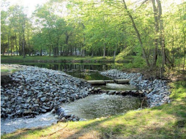
A view of the top of the Crystal Lake Fishway, showing the water control structure (top weir) and two lower stone weirs.
