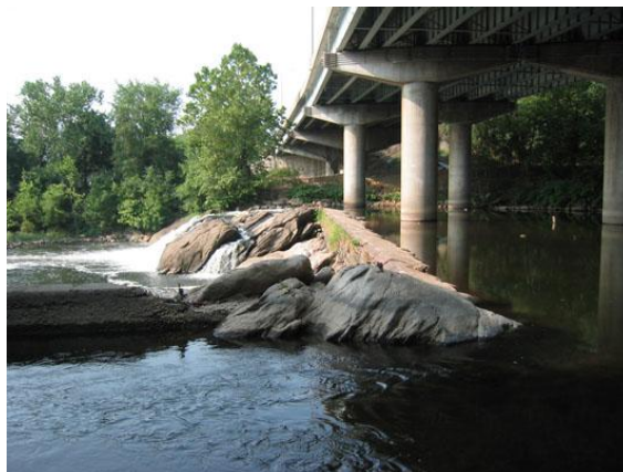
The Tingue Dam on the Naugatuck River, looking south. The Rt. 8 overpass can be seen to the right. The spillway is actually an inch or two higher than the ledge on the far side so during low flows, all spill occurs over the ledge. The future fishway will excavated through the rock underneath the water in the foreground, and proceed northerly toward the camera.
