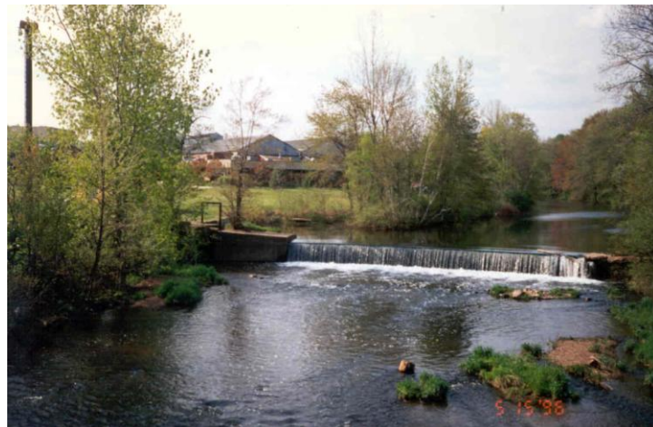
The StanChem Dam- the first dam on the Mattabasset River in East Berlin, CT. The future fishway will be rather U-shaped, circumventing the left end (in the photo).
