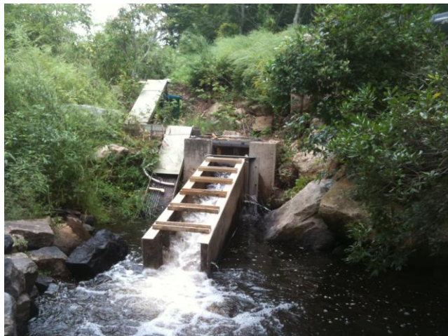
The new entrance of the Mary Steube Fishway in Old Lyme. The old entrance was the concrete structure but the drop was too high for easy entry. The steeppass unit makes it easy for alewives to enter.
