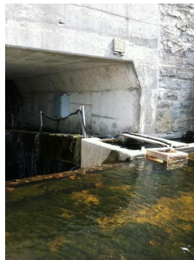
The exit of the Trading Cove Brook Fishway in Montville showing the new counting weir in place. It is the wooden basket-like object attached to the upstream end of the fishway exit. The fishway passes down through a large highway culvert to the left. The dam extends to the left from the exit. The count in the table above represents the first day of operation of this counter.
