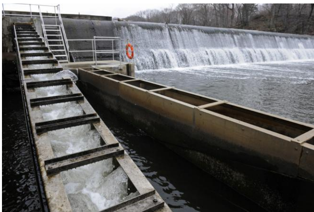
The lower portion of the Mianus Pond fishway in Greenwich, at low tide. The entrance is under the orange life ring. Flow in the upper ramp is coming toward the camera (located at the turn pool) and flow in the lower ramp is flowing away from the camera. (photo by Julie Larson Maher).
