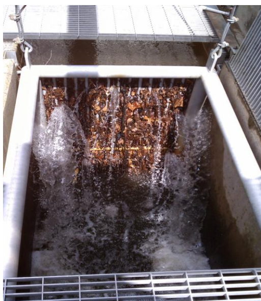
When high flows come, leaves often come with them. This "sorting gate" must be kept down to retain returning adult salmon but it also clogs with leaves, requiring a tedious cleaning.
