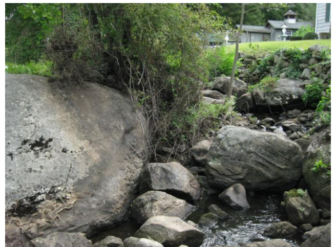
The Wequetequock Pond Dam is not much of a dam. Most of the spillway consists of a very large boulder called Saddle Rock, the eastern third of which is seen in this photo. This photo shows the route of a future stone weir fishway.
