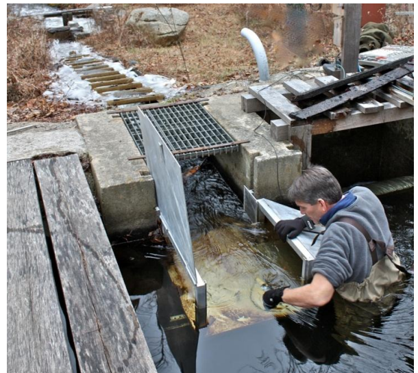
Tim Wildman (CTDEEP- Inland Fisheries Division) installs the camera box outside the exit of the Moulson Pond Fishway. The camera is housed under his right arm and the lid folds down and locks. Images are sent to an instrument box about 50 feet away. There is a removable backdrop that must be cleaned regularly.
