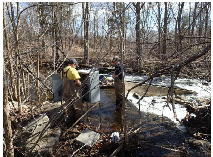
Fish Counter at Landon Dam: Dave Ellis and Bruce Williams (partially obscured by branches) install a fish counter at the Landon Dam fishway.
