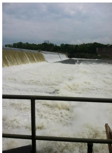
When there is a lot of water pouring over the Holyoke Dam, they cannot operate the fishlift. That is currently the situation. Once the flows drop down to below 40,000 cfs, lifting will begin. Once fish start passing Holyoke, upstream fishways will begin to be opened.
