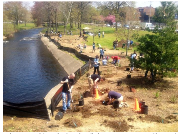
Volunteers and Save the Sound staff planting vegetation in Glenwood Park, Bridgeport. The Apron Fishway is barely visible at the end of the sloping concrete wall. It was high tide and most of the fishway was underwater. The plantings are intended to improve riparian habitat, beautify the site, and discourage geese—not to discourage anglers or visitors as a local newspaper erroneously reported.
