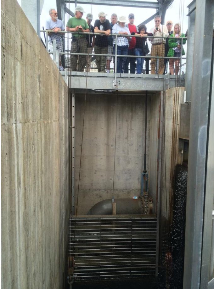
Part of the people in the progressive tour watching the Greenville Fishlift coming up . The cables on each wall lead down to the hopper, which is still underwater. The grate in the back is where the attraction water comes from. The fish will be dumped through the gate at the upper right (photo Sally Harold, TNC).
