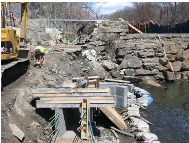
Work proceeds on a steep pass fishway at the 182 nd Street Dam, the first on the Bronx River in NYC. This photo showing the fishway entrance below and the gap in the dam above for the entrance was taken in April.
