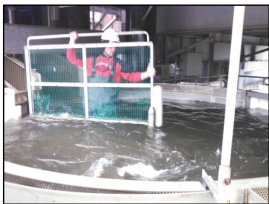
A worker at the Holyoke Dam Fishlift installs a crowding fence in a holding tank to push captured shad into an adjacent tank. This system is used to truck shad from the Connecticut River to other locations.
