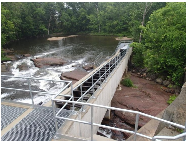
This is the Manhan River Fishway in Easthampton, MA. The photo was taken from the exit looking down. Just before the cover grating begins is a resting pool. Then there is a turn pool. The lower baffled ramp is out of site behind the wall. You can see the entrance pool along with the attraction water gallery at the lower level surrounded by railing.
