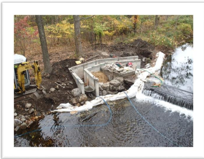
Newmans Fishway under construction. The right-bank pool-and-weir wraps around the end of the two-foot high spillway. A rock retaining wall can be seen between the fishway entrance and the spillway. The entire face of the fishway was backfilled with boulders to hide the concrete.
