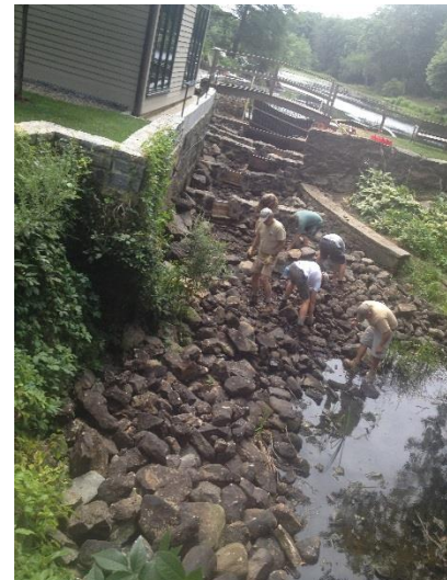
The crew picking rocks for the last weir in the de-watered channel.
