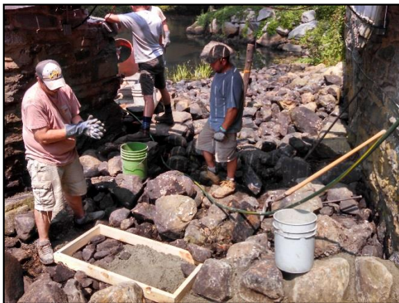
The Tiley-Pratt Dam has two spillways and channels that convey flow down to the stream below the dam. The eastern one was confined in between rock walls and was full of randomly piled rocks. In this photo, the work crew is forming a base for a concrete pedestal to accept weirboards. A full stone weir was built around this pair of pedestals.
