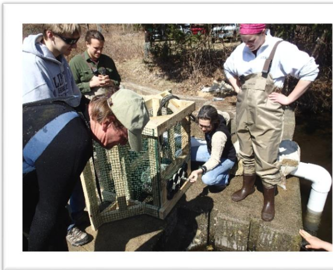
A joint DEEP-TNC work team preparing a new fish counting weir before lowering into place at the Wood Dam Fishway on the Saugatuck River. Sally Harold of TNC applies epoxy foam between PVC pipes. When cured, the foam will prevent fish from wedging themselves between the pipes and force them to pass through the pipe where they will be counted.
