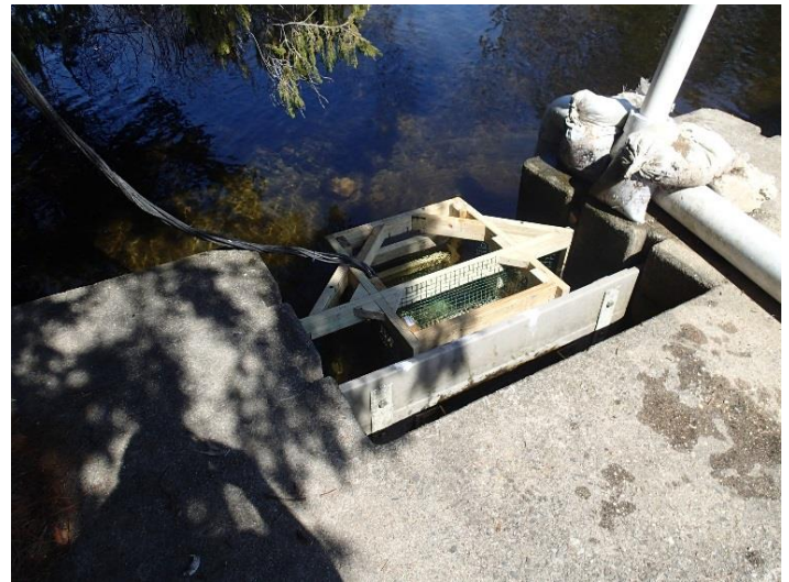
The fish counter weir in place at the exit of the steppass fishway. The cables send the electrical signals from the PVC pipes in the weir to the electronic counter in a nearby lockbox. The white pipe to the right is part of an auxiliary attraction water system (siphon). A Delaware style eel pass is just off photo to the right, also installed on this day.
