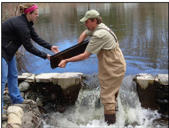
Steve Gephard removes a headboard from the Dorr's Mill Dam Fishway, Saugatuck River, and hands it to seasonal worker Hillary Clifton, allowing water to pass down the fishway. There are two fishways at this dam, this one at the spillway and another that circumvents the dam to the west. Both were TNC projects completed a few years ago with DEEP assistance. This fishway is immediately upstream of the Doc Skerlick Trout Management Area.
