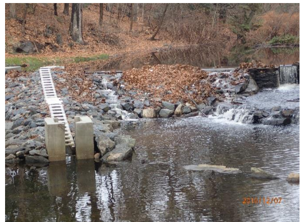
The Upper Pond Dam Fishway at high tide. To the right is the spillway where there is an eel pass.
