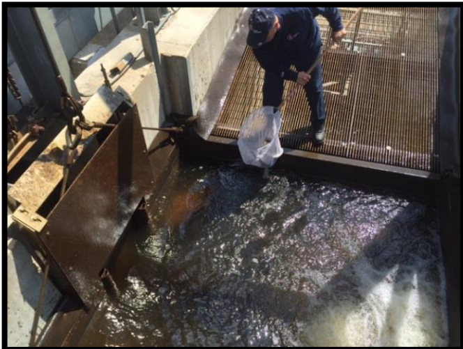
Norwich Public Utilities nets shad out of the Greenville Fishlift hopper and puts them in a truck and transports them above upstream dams to accelerate the restoration process. The worker is standing on the grate, which crowds fish into the hopper as it is raised. The water and fish are discharged out the gate to the left normally but the hopper is held up while workers net out fish.
