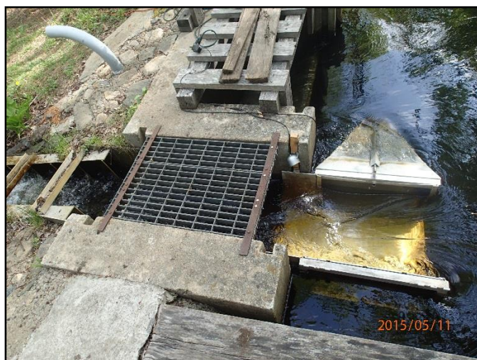
After fish move through the pool-and-weirs at Moulson Pond, they ascend a section of steppass fishway and then pass through the camera box (lid off). The camera is at the end of the far triangular section. Nine shad have come up this fishway so far.
