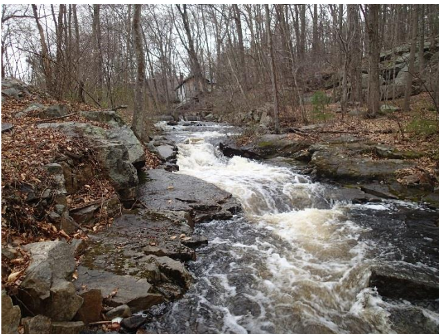
Believe it or not, this is a constructed fishway. Tons of rock were brought into to build a series of pools and cascades that alewives can surmount in this nature-like Lower Guilford Lake Fishway (East River, Guilford). Alewives have used it each year since its construction and this year over 2,000 have climbed it to enter the pond.
