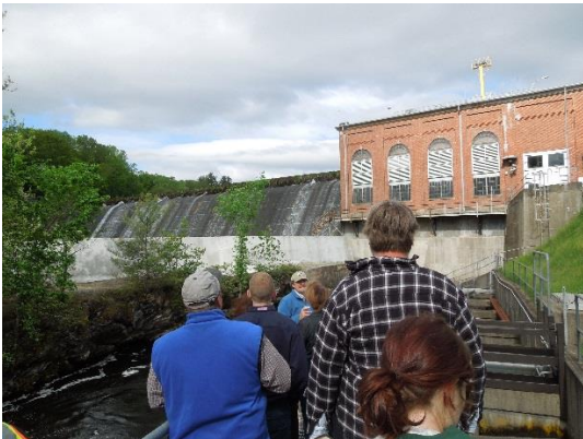
Tour of the Rainbow Dam and Fishway, May 20, 2015.
