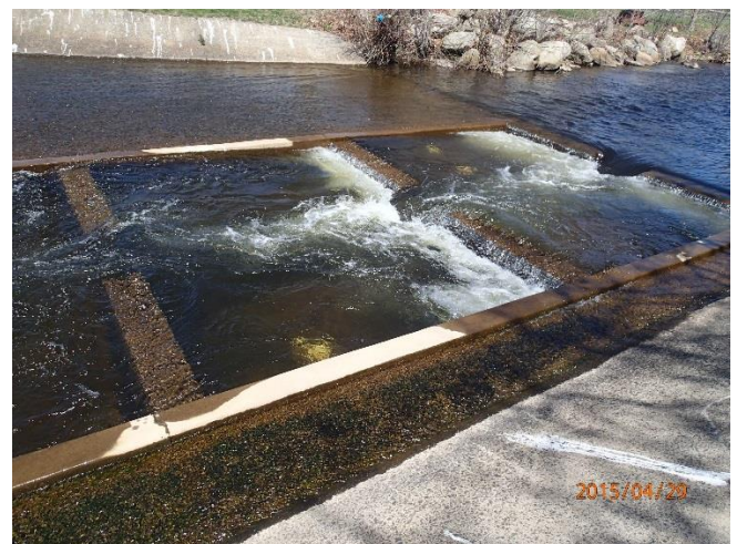
Another photo of the Pequonnock Apron Fishway, showing the nice plume of water shooting through the notches in the weirs. The lowermost weir is underwater and not critical to the fish at this tide. But at lower tidal stages, that weir is exposed like the upper two are in this photo and it is helpful for allowing fish to get upstream.
