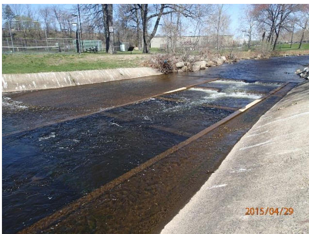
The Pequonnock Apron Fishway is a series of pools recessed down into the concrete apron that was constructed across the river decades earlier. The pools are separated by concrete weirs with a notch in them. The fishway provides adequate depth of water for fish to migrate. The water in the fishway is 2 – 3 feet deep. The water outside the fishway is 2 – 3 inches deep.
