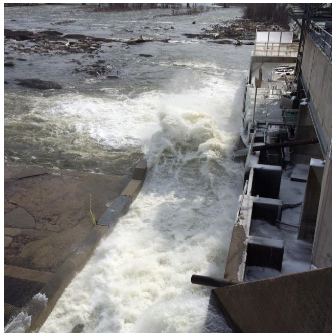
This is right below the Holyoke Dam. If you look just to the right of the huge wave, you'll see a concrete wall. That is the location of the entrance to the spillway fishlift. There is a lip at the bottom of the spillway apron that sends the water from the bypass shooting into the air and creates a calmer zone underneath where migrating fish can swim and find the entrance.
