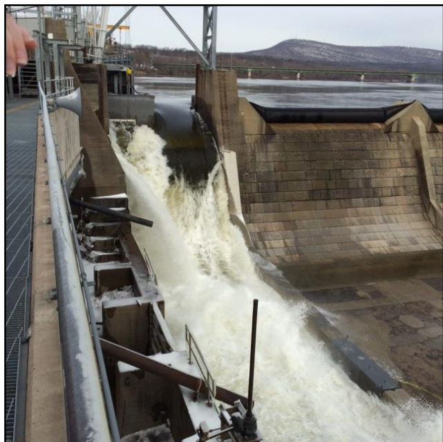
The new downstream bypass at Holyoke Dam. The main chute resembles what was there previously but to the left are a couple of submerged openings that attract and pass down-running species that don't favor the water surface, like sturgeon and silver-phase American Eels. All go down the chute. To see where they end up, look at the next photo.
