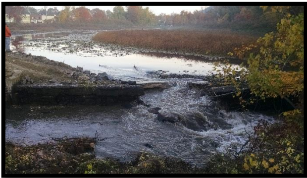
The first breach of Pond Lily Dam looking north to south.
