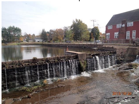
The Broad Brook Dam (shown here last summer) was in need of repair. A Delaware style eel pass was added during the winter repairs. Note that the top of the dam has wooden flashboards.
