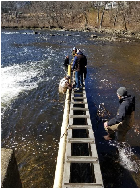
Attaching the attraction water pipe at Wood Dam, Saugatuck River. In back in wetsuit S. Gephard, with blue hat Tim Wildman, in water with waders Bruce Williams, on fishway with back to camera Dave Ellis, foreground, seasonal worker Peter Grundy.
