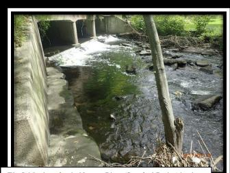
The I-95 culvert for the Noroton River (Stamford-Darien) has been perched and blocking river herring runs at most tide stages. Plus the flow is shallow and fast in the long culvert.
