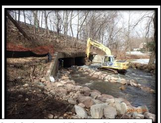
Save the Sound got grants to build a rock ramp fishway at the lip and install off-set baffles inside the culvert. This work is just now finishing and the fishway will be a featured event for World Fish Migration Day on Saturday. Designed by Princeton Hydro; constructed by Schumack Construction.
