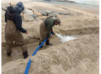
Dave Ellis (right) with seasonal worker Peter Grundy uses a gas-powered water pump to try to blast a channel through the Rocky Neck beach to allow Bride Brook to flow to Long Island Sound. The channel where they are standing is normally three feet deeper and lined with rocks.
