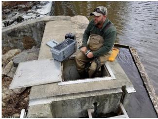
Dave Ellis installing the electronic fish counter into the locked cabinet at the Branford Water Supply Pond Fishway on Queach Brook in Branford.
