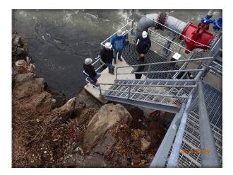
The entrance of the fishlift at river level below. The water enters the river below the person with the blue jacket. The large pipe delivers extra attraction water to the fishway.
