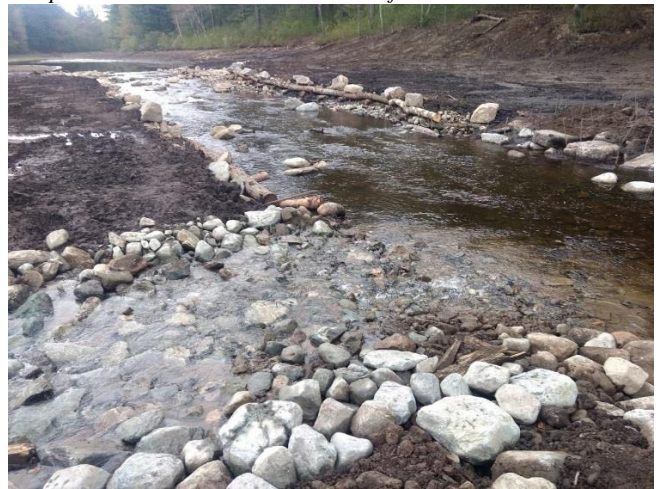
The newly restored stream channel with a small tributary from Blackledge Falls entering from the left in the foreground. By looking at the edge of the woods in the background, you can see where the pond was.
