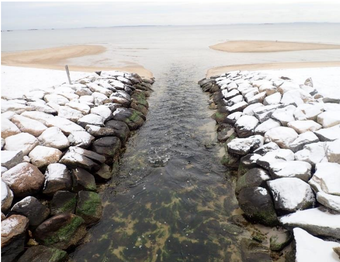
In past years, winter storms sometime push tons of sand up on the Rocky Neck State Park beach where Bride Brook enters Long Island Sound. This makes us go out and dig it out so Alewives can come in and spawn. This year, the entrance looks great with no issues for incoming Alewives. Replacing the old rusty pipes with this new channel was a Save the Sound project several years ago.
