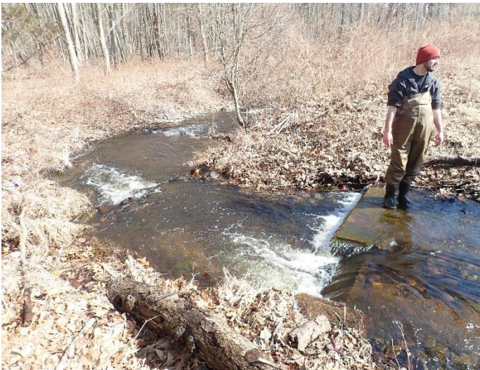
The beaver are gone from Crystal Lake in Old Saybrook so seasonal Matt Augusto and crew tuned up that Town-owned nature-like fishway. Fish that pass through the Fishing Brook Fishway can swim up another mile or so and enter Crystal Lake via this fishway.
