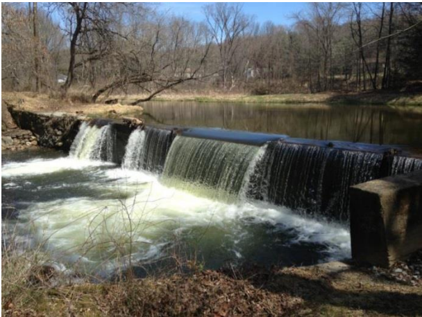
Old Papermill Pond Dam before. The spilling water hides the heavily degraded condition of the dam. This springtime photo shows a full pond.
