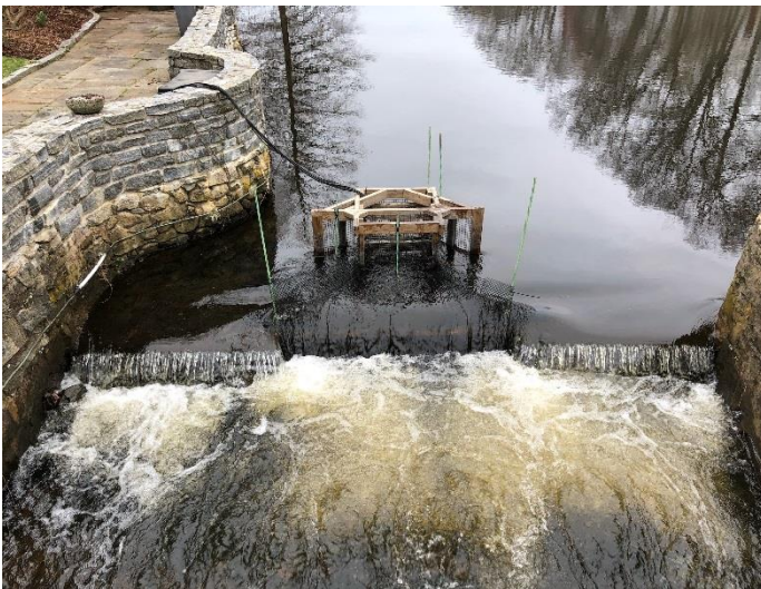
The Tiley-Pratt Fishway on the Falls River in Essex was built several years ago at a private residence. It is the first dam on the Connecticut River tributary and for the first time we've installed an electronic fish counter at the top, thanks to the cooperation of the property owner. Two more fishways will be built upstream this summer.
