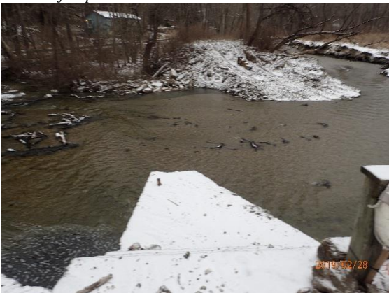
Old Papermill Pond Dam before. The spilling water hides the heavily degraded condition of the dam. This springtime photo shows a full pond.
