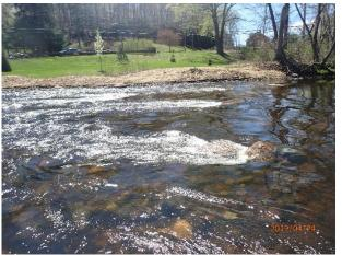
The same site after pipe removal. Boulders were placed in the stream to help guide flows and to provide velocity blocks for migrating fish. They were spaced to reduce conflicts with paddlers.
