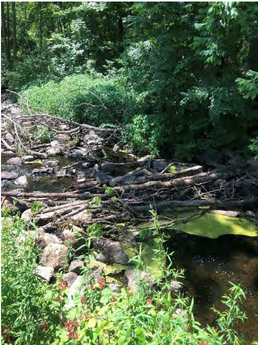
The bypass reach at the Branford Supply Pond Dam, clogged with debris, discouraging downstream passage.
