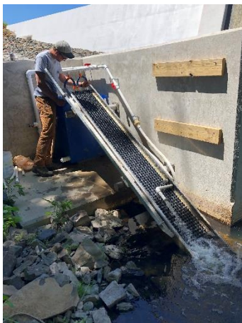
Kevin Job adjusts the flow of the new Kensington Pond Dam Eel pass on the Mattabesset River as Tim Wildman takes the photo. The hinged predator cover is opened to the left for the photo.
