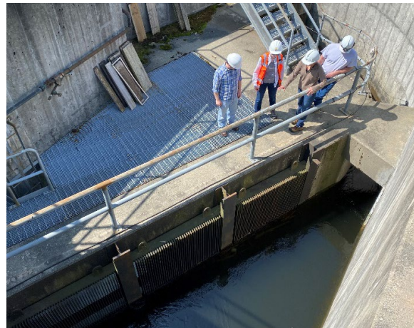
The exit of the Vernon Fish Ladder. Jen Griffin (GRH) and agency staff are standing on where attraction water system is located (to maintain desired velocities and flow vectors).
