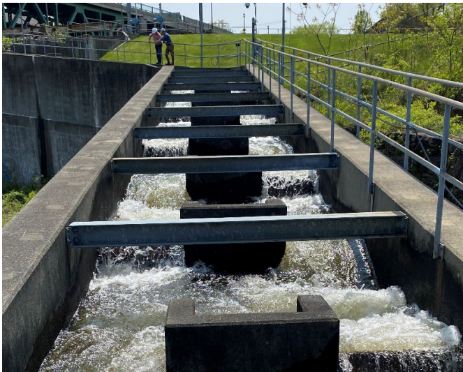
The Turners Fall Spillway Fish Ladder (at the dam), an Ice Harbor design, with alternating baffles inserted for the weirs to improve passage performance. Engineers and Steve Leach (FLP) shown by a turn pool.
